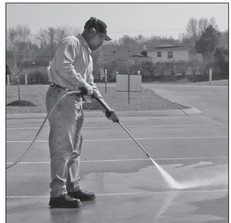
Figure 19 - Optimum angle to cleaning surface
